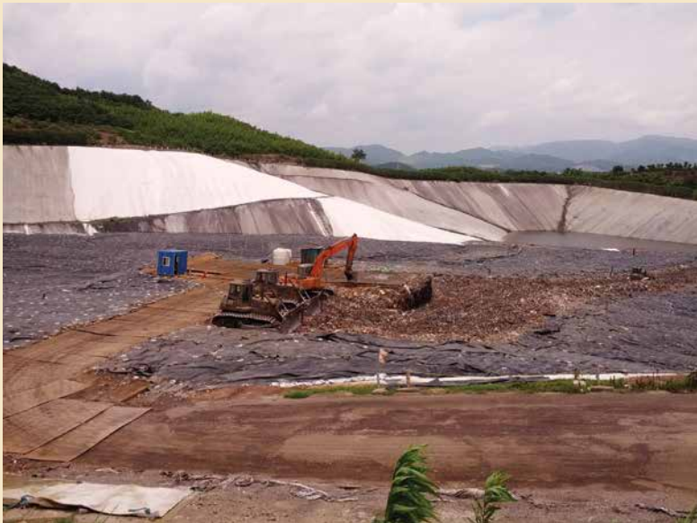
Photo 3.1 Landfill in China
